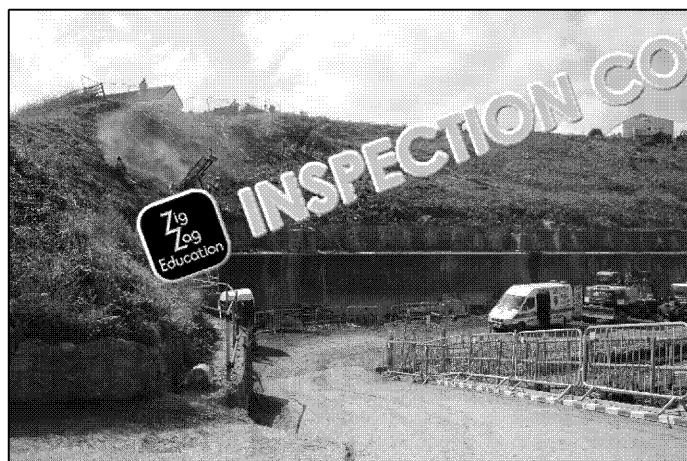
Figure 15: Soil nailing in East Cliff
