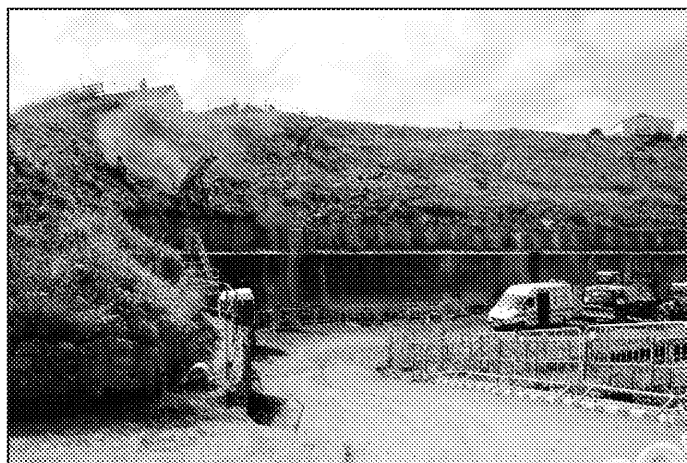
Figure 15: Soil nailing in East Cliff
