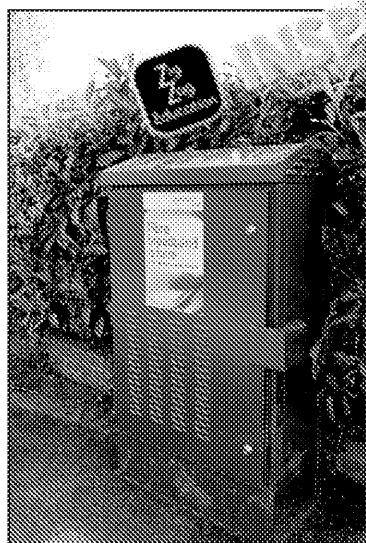
A modern street cabinet using FTTC
